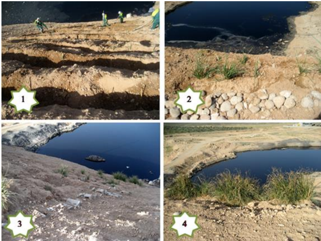
Figure 2. Vetiver planted on terraces around leachate ponds, at planting (1) and at 4 months old (4)
