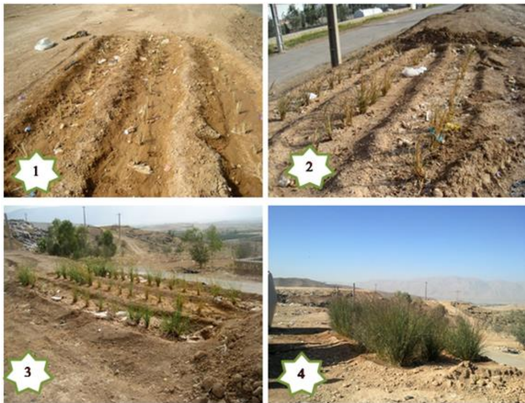
Figure 3. Vetiver planting on top of a completed cell, at planting (1) and at 4 months old (4)
